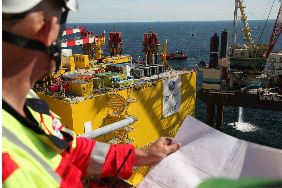
Figure 4: DolWin Gamma installations
