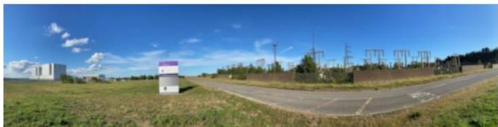
Figure 2: Photos taken on 20 June 2020 of the redundant Bradwell substation.
